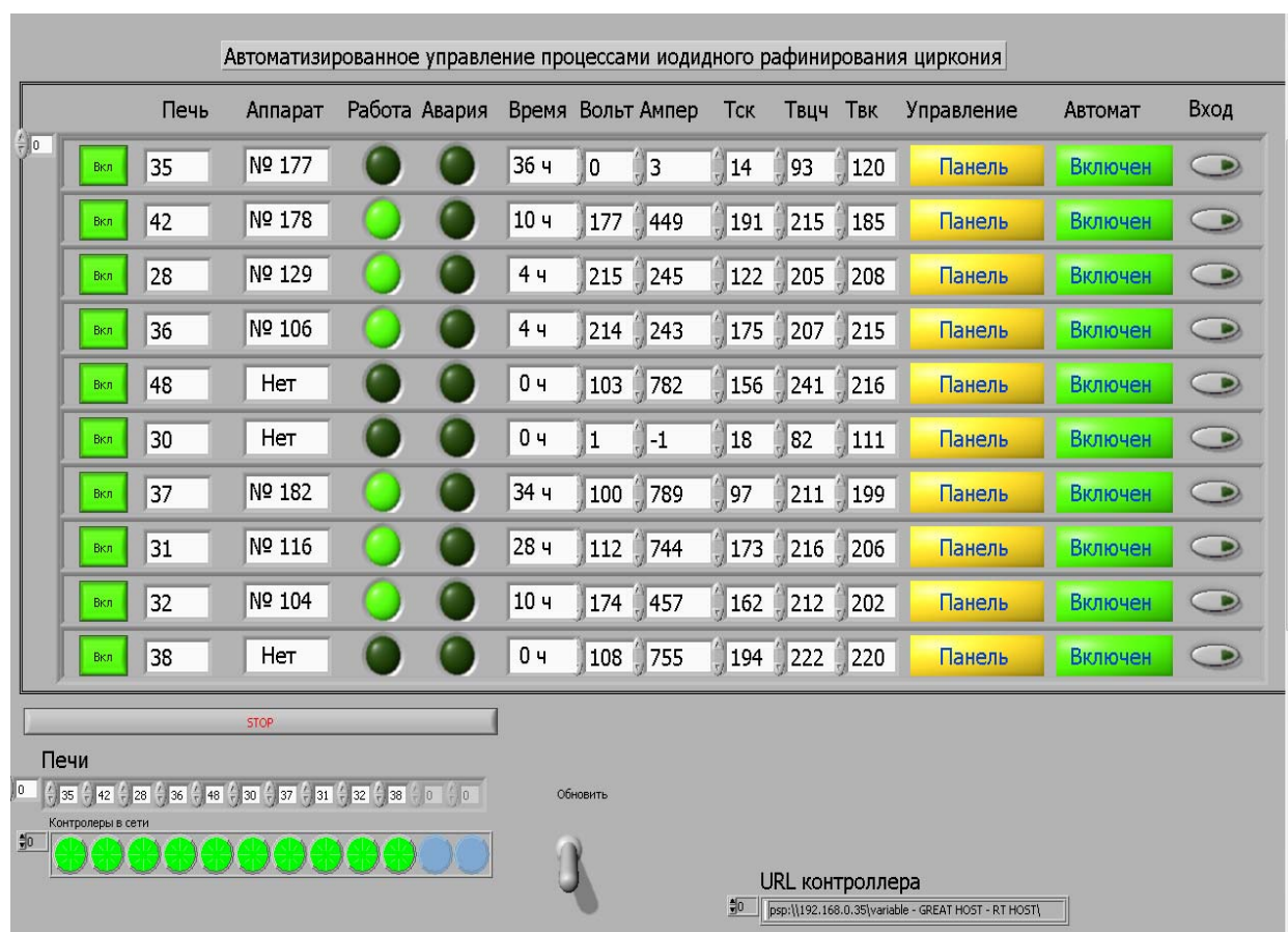
Fig. 8. The front panel of the supervisor on the computer to monitor the course of the process
