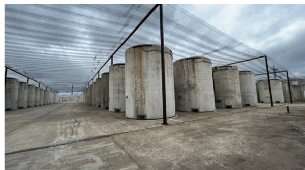
Fig. 2. Dry container-type spent-fuel storage facility at the ZNPP
