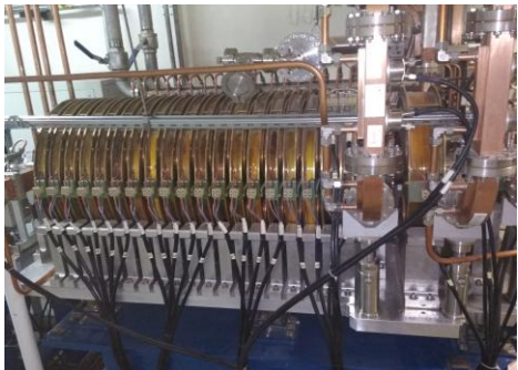
Fig. 3. The view of installed accelerator solenoids
