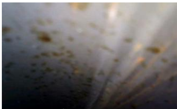
Fig. 3. Photo of the inner surface of the pipe below the impeller at the turn
