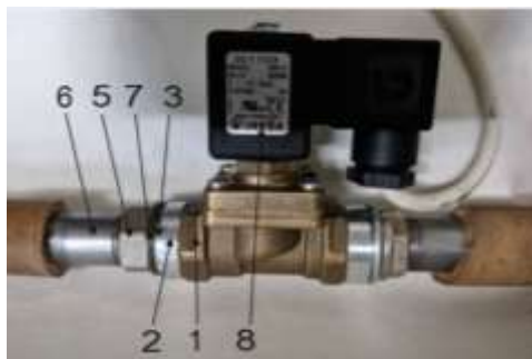
Fig. 6. Emergency valve with 2 copies of created vacuum connection: 1 – standard valve body; 2 – restrictive ring; 3 – half rings; 5 – clamp nut; 6 – threaded pipe; 7 – intermediate washer; 8 – electromagnetic valve control
