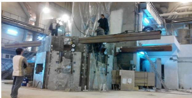
Fig. 11. Biological shield of the NSC KIPT SCA "Neutron Source" core without top movable lid-parts
