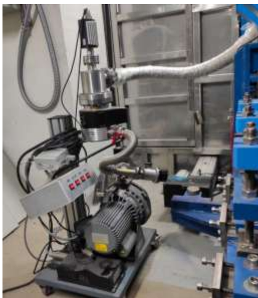
Fig. 12. The preliminary pumping unit in operation
